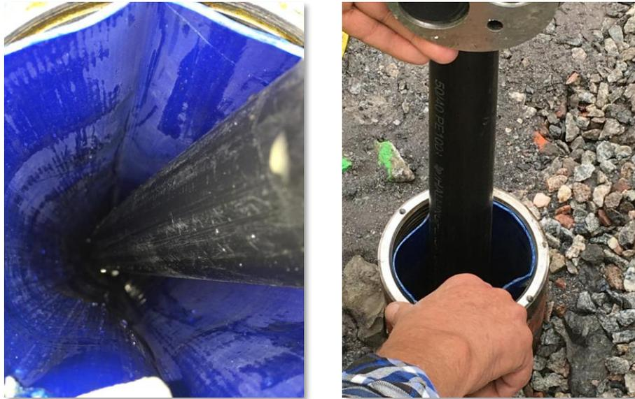
Figure 4. Pictures of the coaxial borehole heat exchanger during installation. Pictures: Patricia Monzó.
