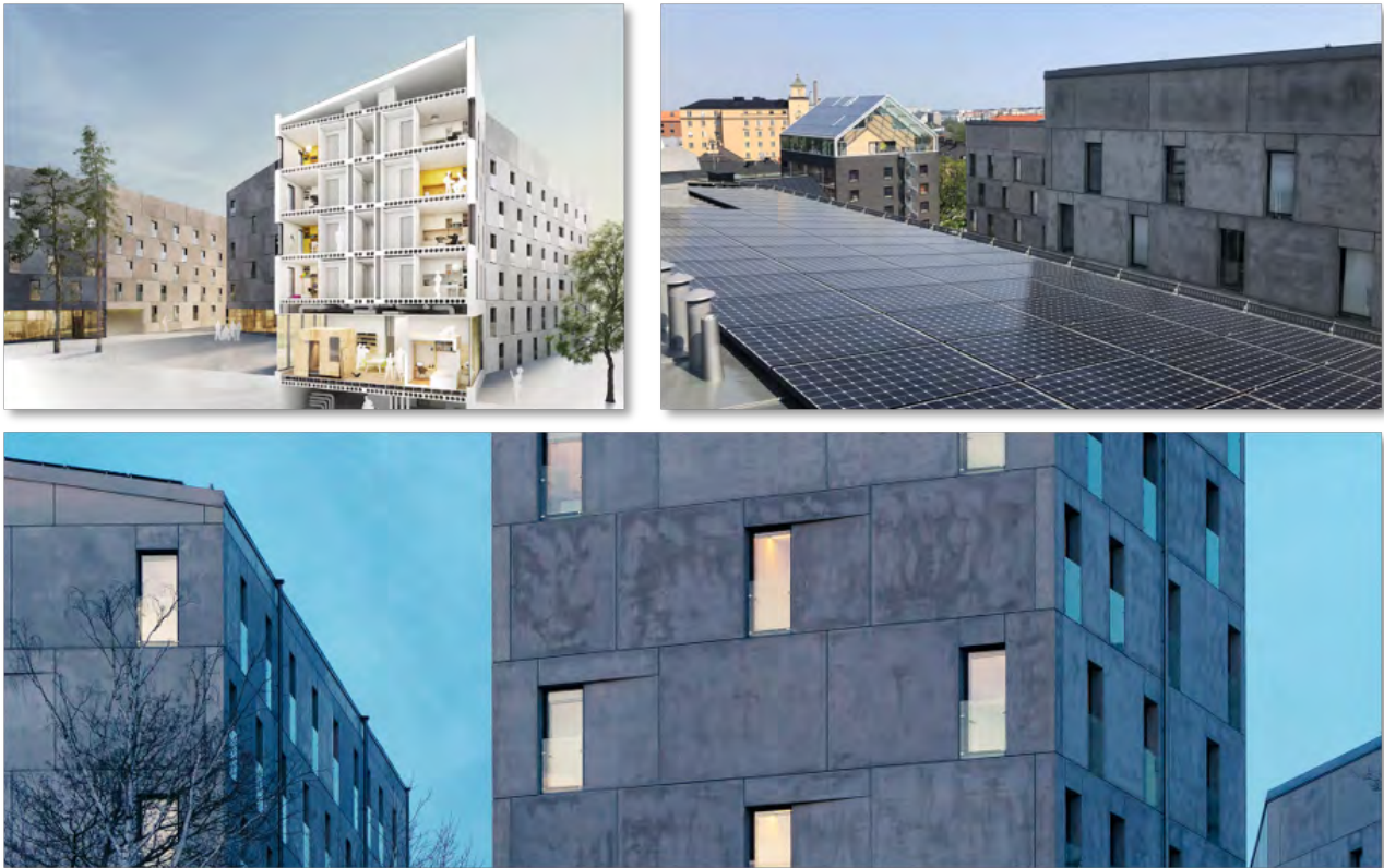
Figure 5.1: Photos and illustration of the three buildings in Forskningsen 2. Illustration: Semrén & Månsson. Pictures: KTH Live-In Lab.
